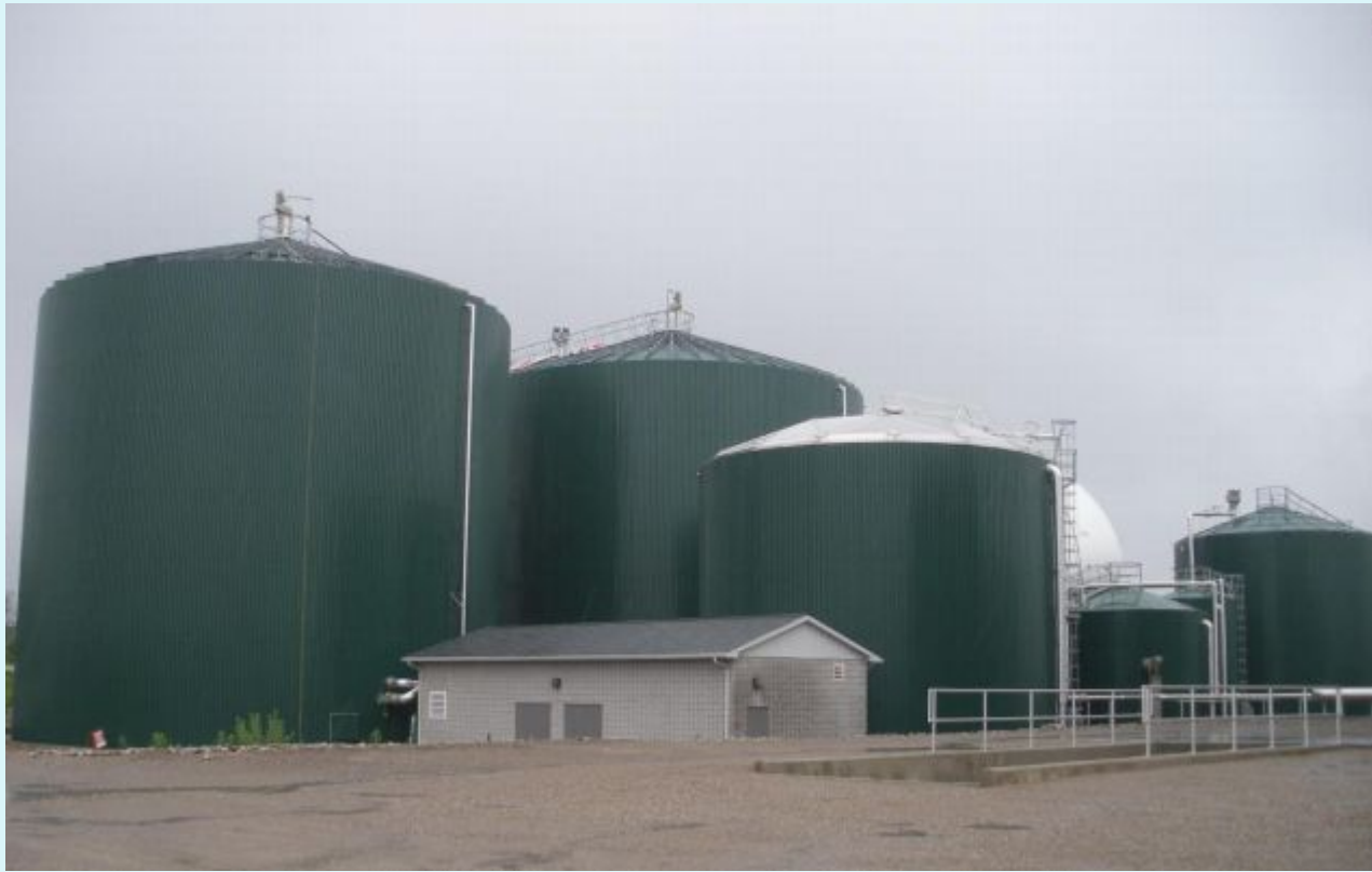
Anaerobic Digesters and Reception Tanks
